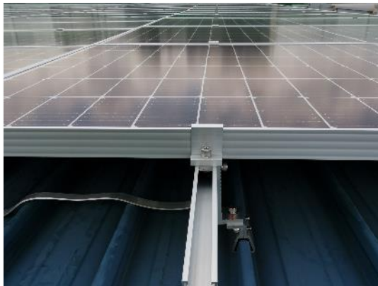
Module mounted with sufficient ventilation
