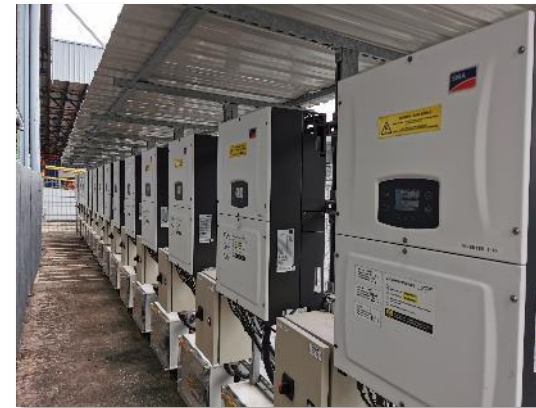
PV inverters mounting with ventilation
