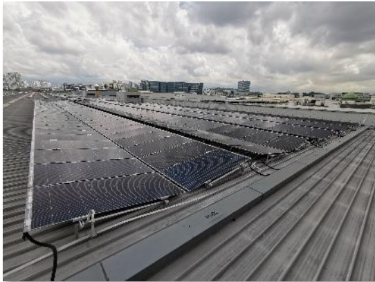
DC cables on cable trays
